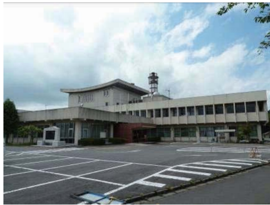
Photo 6.3-17 Appearance of damaged building (Kasama city)
