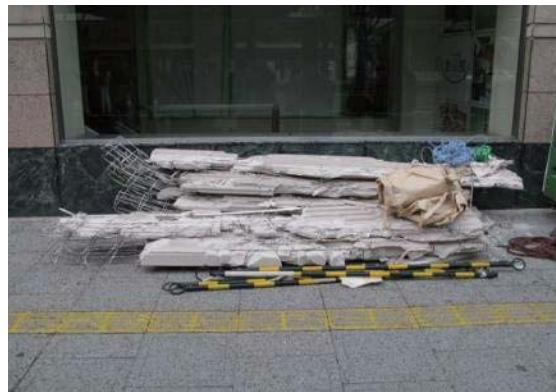
Photo 6.3-48 Dropped AAC panels
