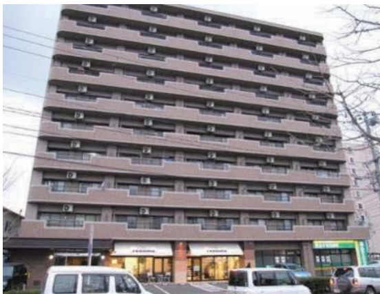
Photo 6.3-41 Appearance of damaged building (Aoba ward, Sendai city)
