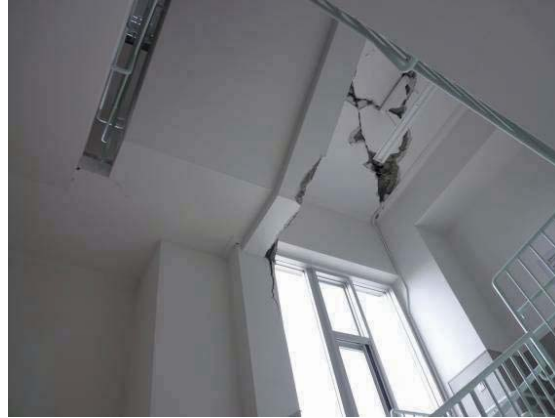
Photo 6.3-36 Bottom of the tower
