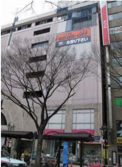
Photo 6.3-47 Damaged building with AAC panels (Aoba ward, Sendai city)
