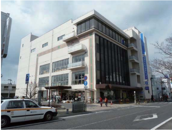
Photo 6.3-39 Appearance of damaged building (Sukagawa city)
