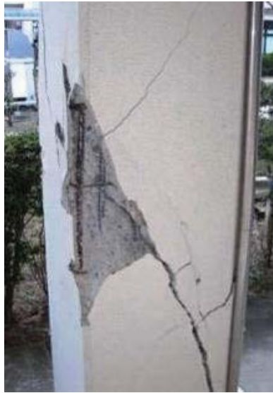
Photo 6.3-13 Shear cracks of first-story columns
