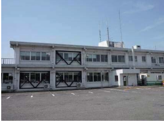
Photo 6.3-37 Appearance of damaged building (Hitachiomiya city)
