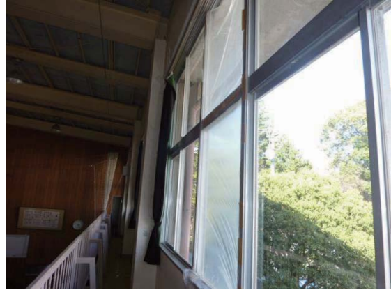
Photo 6.6-10 Breakage of window glasses installed to fixed window frame with glazing bead
