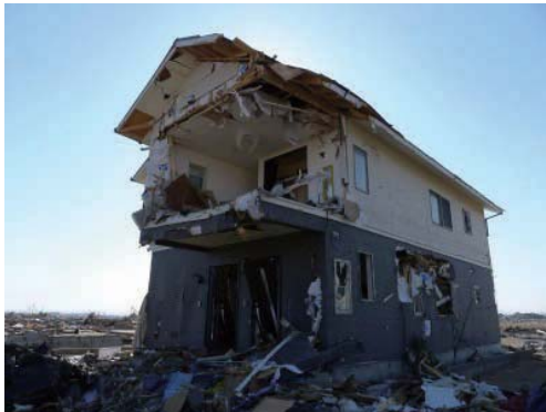
Photo 7.4-9. Remained house which didn't have survived buildings in the direction where the tsunami came in Arahama-shin, Wakabayashi ward, Sendai city.
