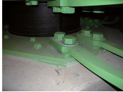
Photo 9.2-22 Peeling off of paint and loose of the bolts of U-shaped steel dampers
