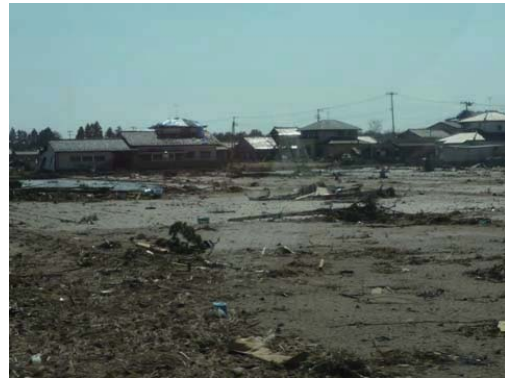
Photo.7.4-6. Many wood houses remained.
