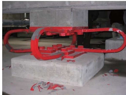
Photo 9.2-16 U-shaped steel damper
