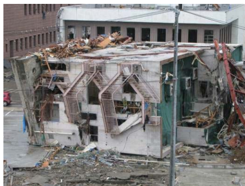
Photo 7.2-9 Overturning of a 3-story steel building
