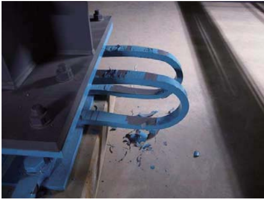
Photo 9.2-22 Peeling off of paint and loose of the bolts of U-shaped steel dampers
