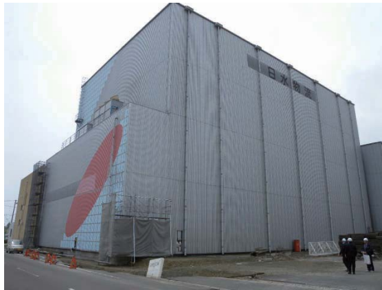
Photo 9.2-5 SI building (B) – Steel warehouse -
