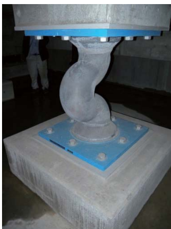
Photo 9.2-17 Lead damper and cracks on the surface
