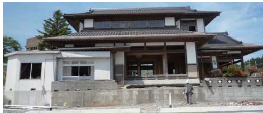
Photo 7.4-29. Japanese traditional wood house (5) which was not carried away under about 5 m water depth in Akasaki-cho, Oofunato city.
