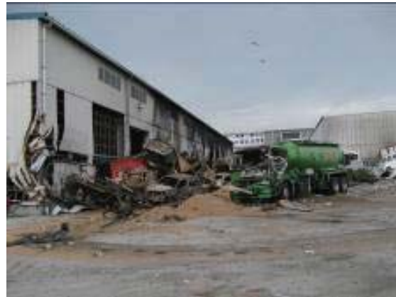
Photo 8.2-2 Tsunami fire at a port warehouse (Sendai city, Miyagi prefecture)
