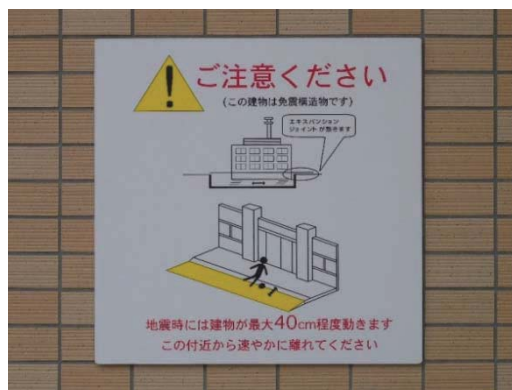
(b) Sign board to warn about seismic gap
