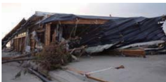
Photo 7.4-22. Glulam frame structure remained in Arahama, Watari town.
