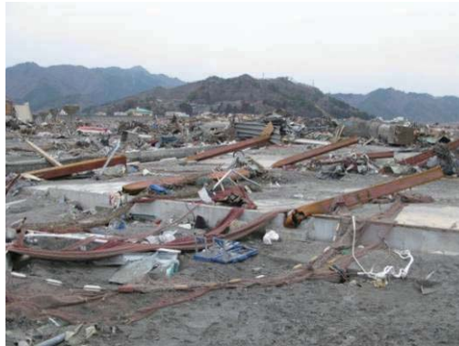
Photo 7.2-8 First-floor columns falling in the same direction
