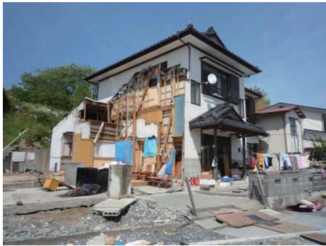
Photo 7.4-27. Wood house (1) remained under the water depth of over 7 m in Akasaki-cho, Oofunato city.
