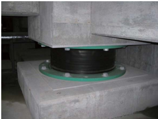
Photo 9.2-15 Natural rubber bearing
