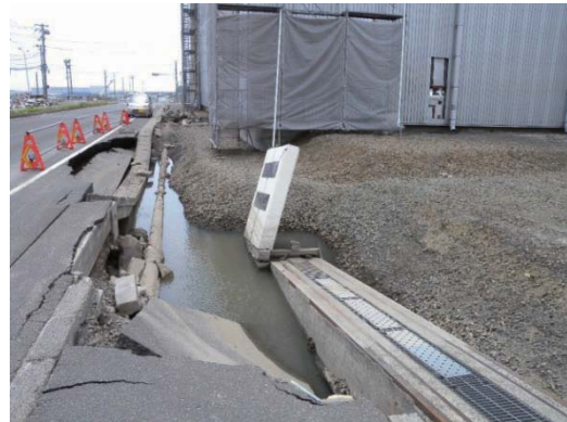
Photo 9.2-9 Excavation of ground
