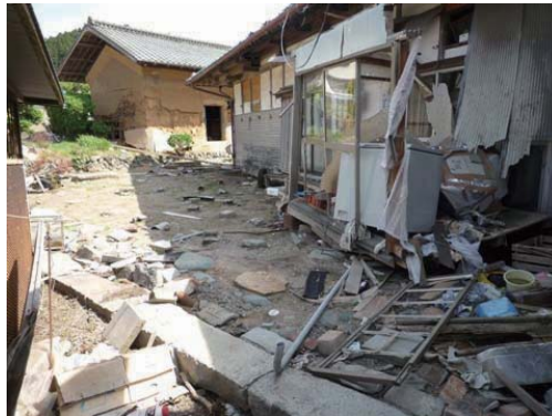
Photo 7.4-33. Survived old house (12) which rotated and moved horizontally in Akasaki-cho, Oofunato city.
