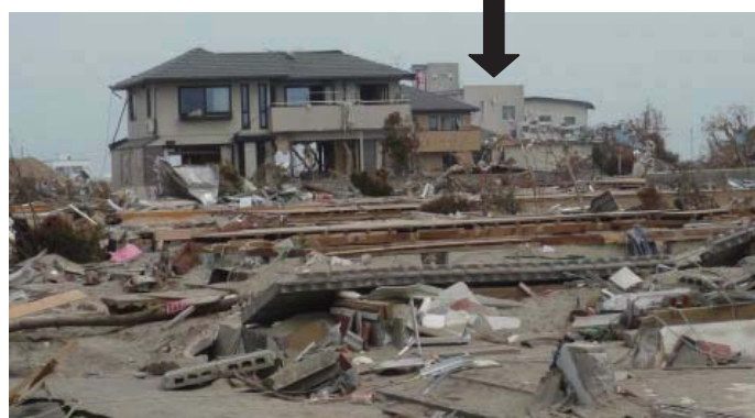
Photo 7.4-21. Wood houses (15) which were not washed away selectively in the downstream of a factory building.
