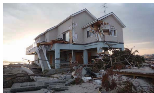
Photo 7.4-23. Mixed structure which has 1 st story of RC structure and wooden 2 nd story.
