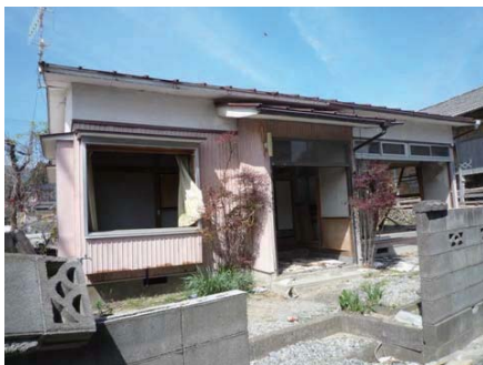
Photo 7.4-31. Survived house (9) which seemed to have comparatively slight structural specifications in Akasaki-cho, Oofunato city.
