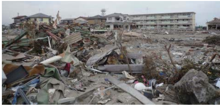
Photo 7.4-20. Group of wood houses (14) which were not washed away in the downstream of a RC apartment house in Yuriage
