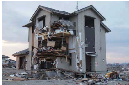
Photo 7.4-25. 3-story wood house remained in the north of Arahama port.
