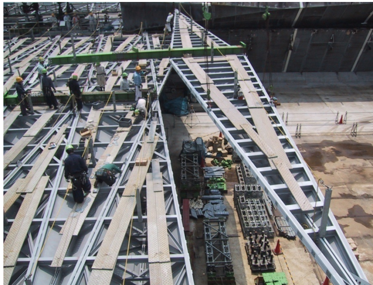
Construction using setting-beam
