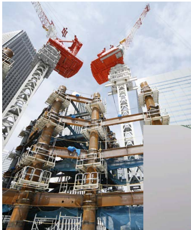
Core zone (Concrete filled steel tube)
