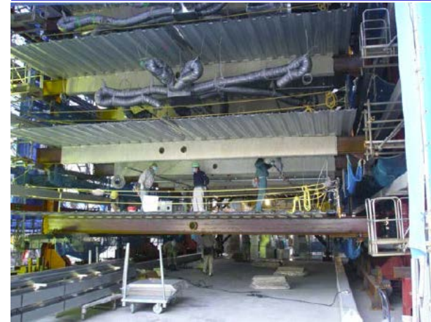
Site Prefabrication System
