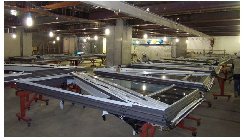
Joint and sealing of curtain-wall units
