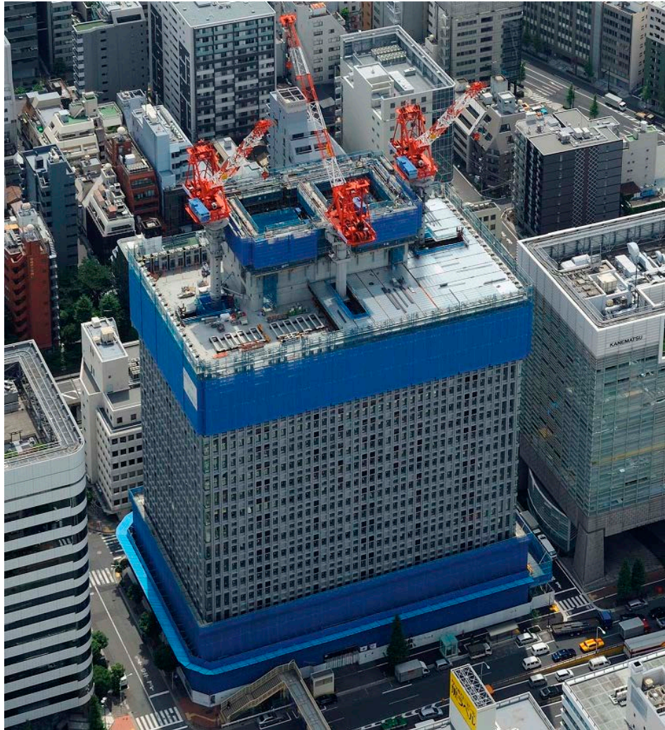
RC core wall + Hybrid perimeter frame
