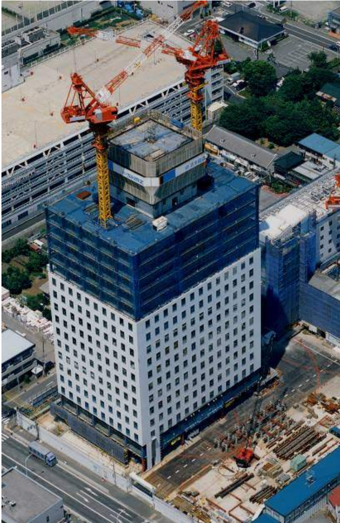
RC core wall + Steel rigid frame
