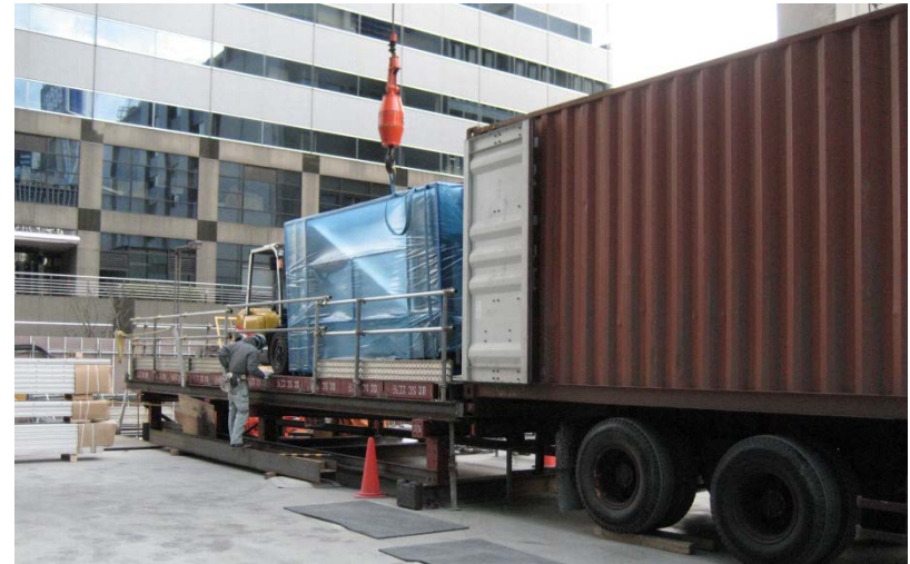
Transportation of curtain-wall components
