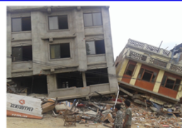
Fig. 1. Soft first story collapse in 2015 Gorkha Earthquake Nepal.
