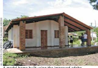
A model home built using the improved adobe construction method
